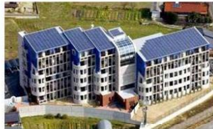
Rented type Eco-Apartment House with Photovoltaic Power Generation, First in Japan
