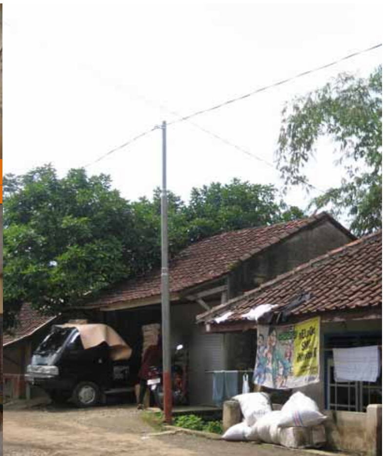
Newly installed electricity grids and polls
