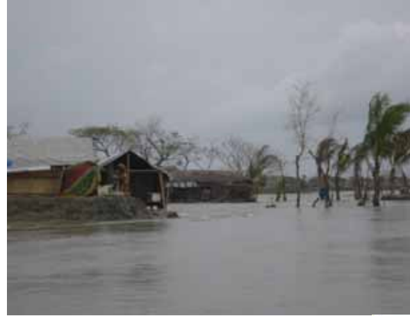
Picture 02: Failure of embankment
