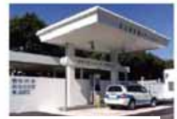
Kitakyushu hydrogen station
