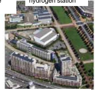
Photovoltaic generation panels installed on roofs of museum, company dormitory and condo in the Higashida street
