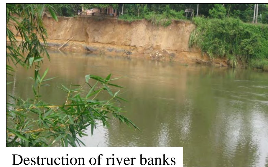
Destruction of river banks
