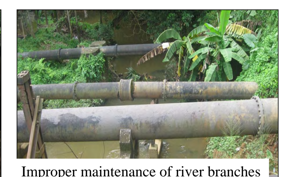
Improper maintenance of river branches
