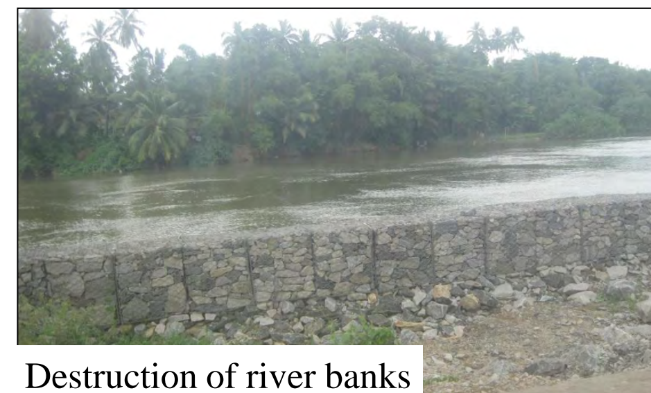
Destruction of river banks
