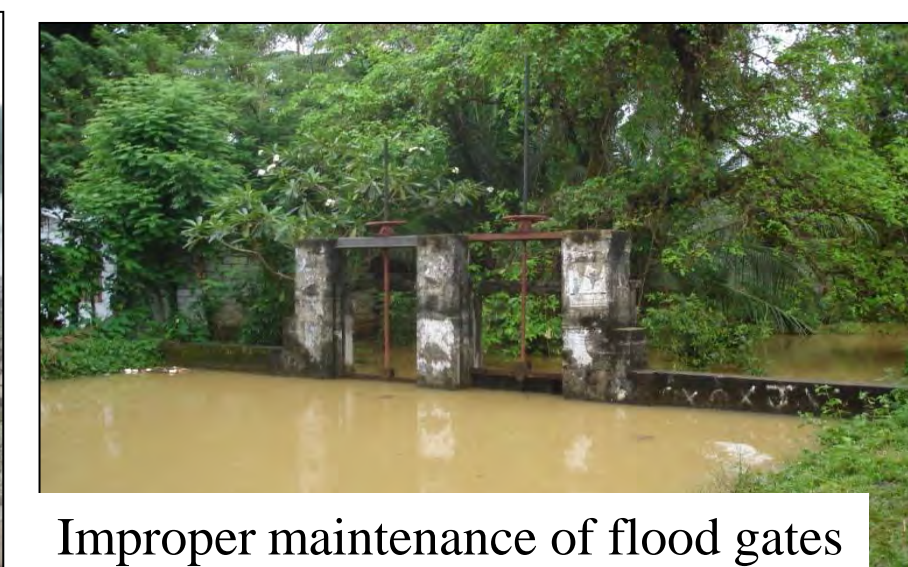
Improper maintenance of flood gates
