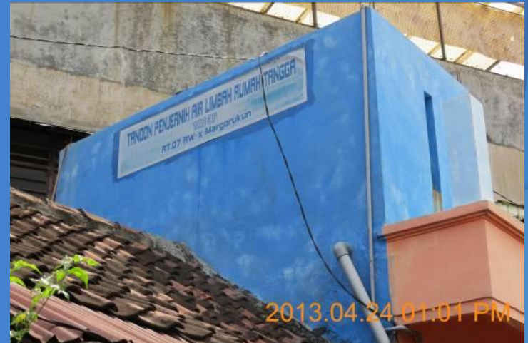
Reservoir WWTP in which there are filters
