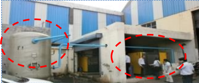
Installation of new receiver and new air compressors (not inverter type)
