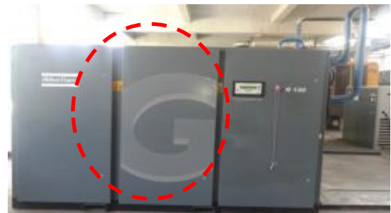
Installation of new receiver and new air compressors (not inverter type)
