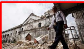
7.2 earthquake toppled centuries-old Sto. Niño church belfry
