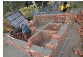
Construction of Pond Sand Filter (PSF) by DDI, an alternative solution for saline water
