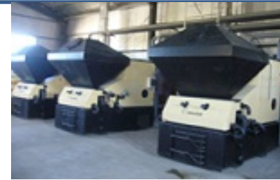
High-efficiency Heat only Boilers, Suuri-Keikaku, Mongolia
