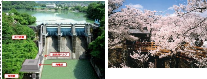
Takato Cherry Blossom Power Plant (Ina City) (Capacity: 180kW, for about 350 households)
