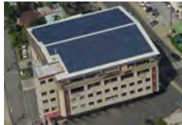
Installing solar PV system, PCKK, Palau Maldives
