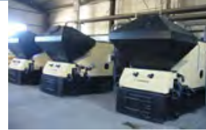
High-efficiency Heat only Boilers, Suuri-Keikaku, Mongolia
