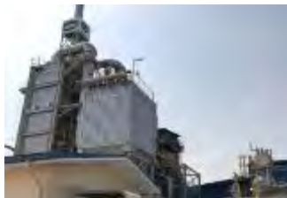
Waste to Energy Plant, JFE engineering, Myanmar
