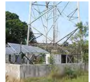
Smart Telecom Towers
