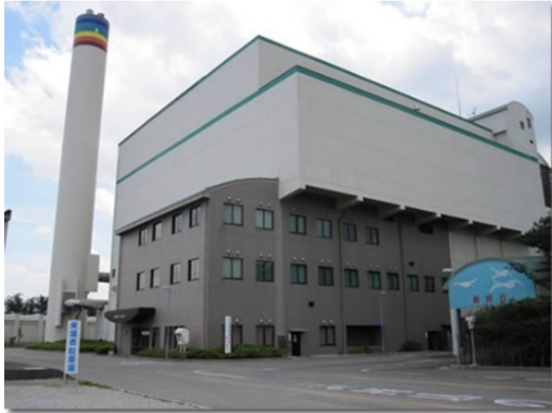
Yonago city clean center (waste-to-energy power generation)
