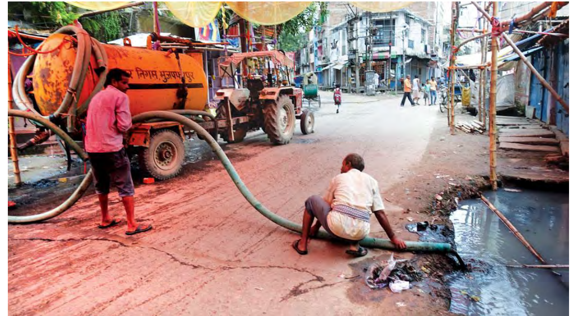
FS being dumped at open drain, India
