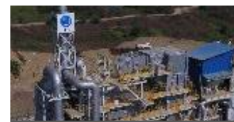
Waste to Energy Plant, JFE engineering, Myanmar
