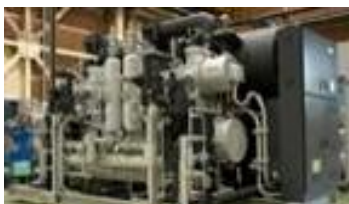
High-efficiency refrigerator, Mayekawa MFG, Indonesia
