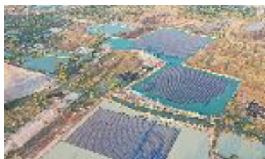
Floating Solar PV, TSB Co., Ltd., Thailand
